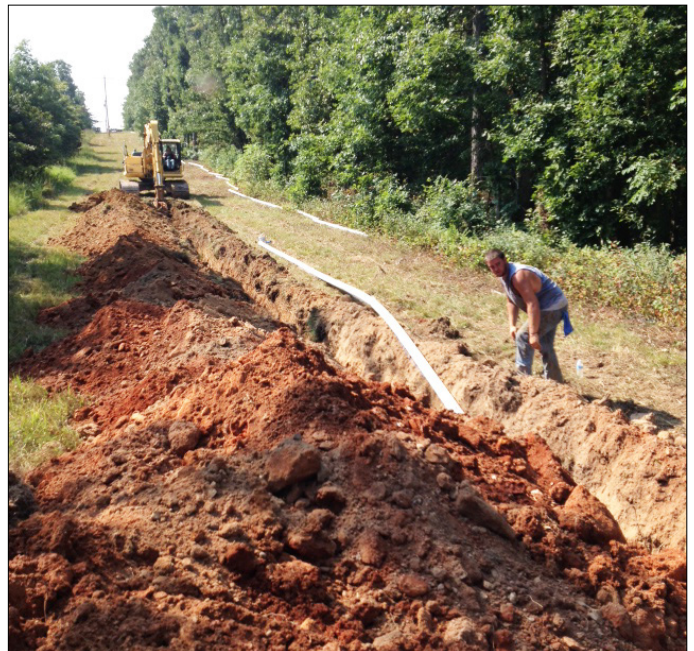
Phelps County Public Water Supply District #1 project (above) while under construction, in the vicinity of Edgar Springs.
